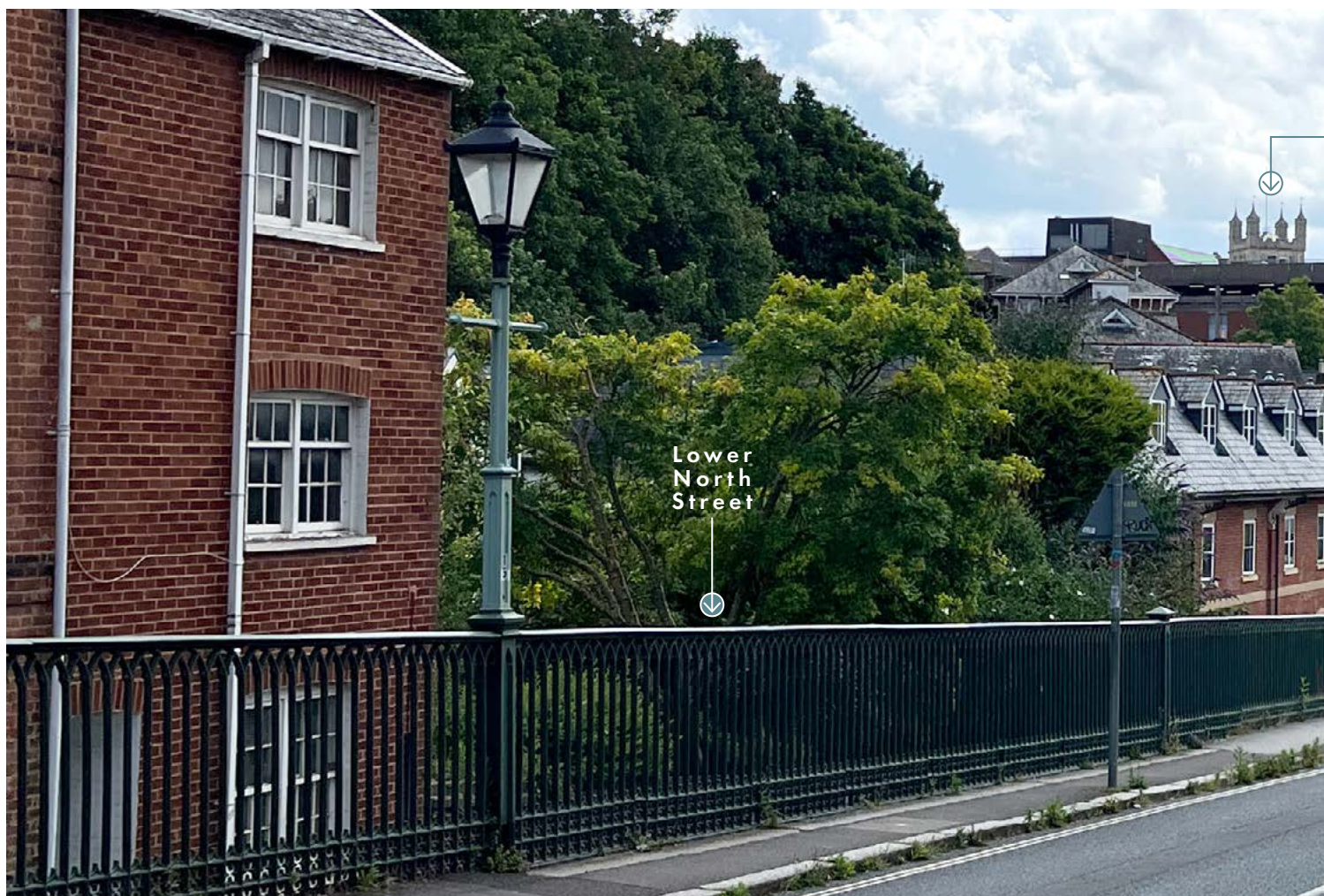
Fig 45 Photo showing A01 St David's Hill / North Street view. Date of photograph: 11 July 2024. Camera: iphone 12
