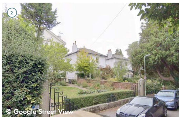
Fig 102 Pennsylvania Crescent was positioned to take advantage of views across the city and to the Cathedral. Site surveys undertaken during the Summer found that the maturing of trees in the foreground of the crescent means ground level views were obscured, but upper floor views may still be possible.
