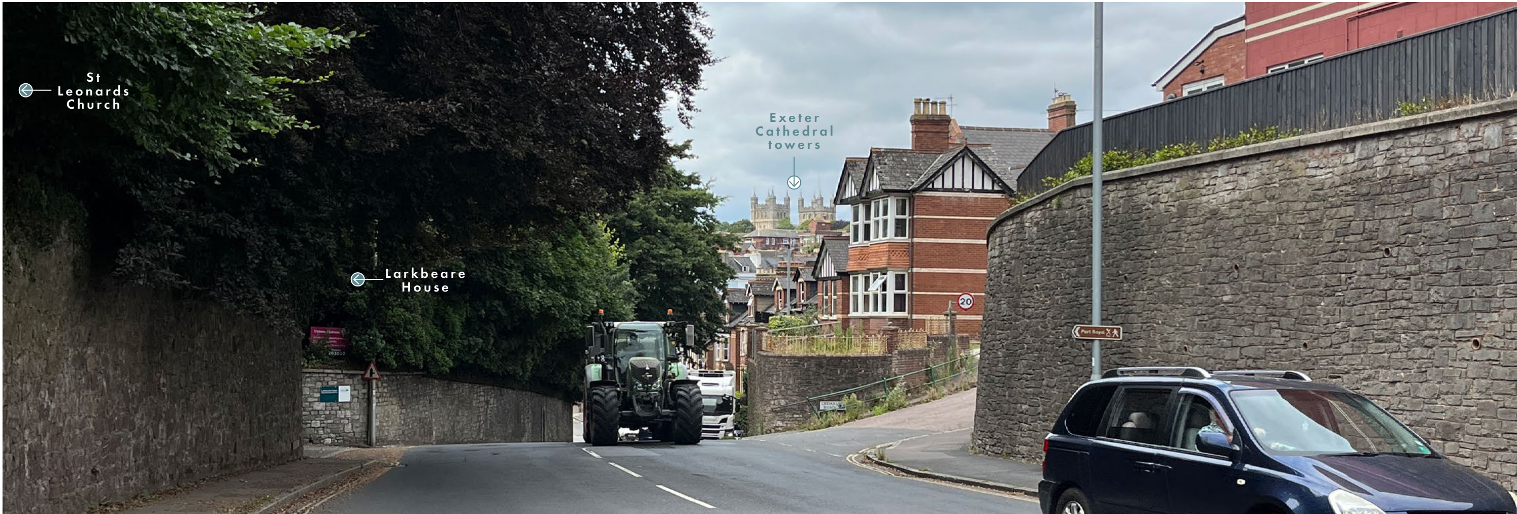
Fig 47 Photo showing A03 Topsham Road view towards Exeter City Centre. Date of photograph: 2 August 2024. Camera: Cybershot Sony RX100 SLR.
