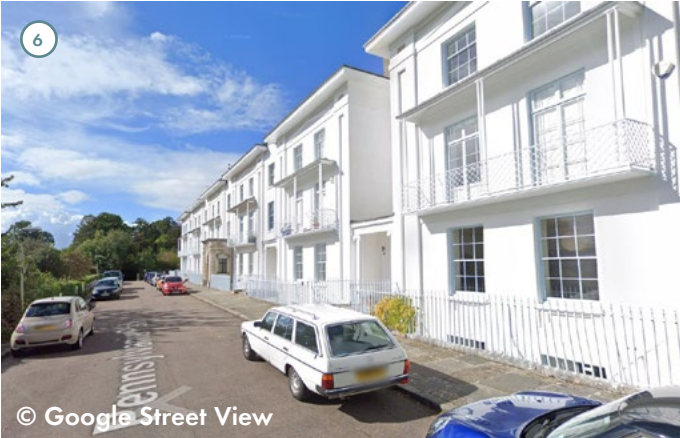
Fig 106 Pennsylvania Park built to take advantages of views from the north across the city. The trees in the garden now obscure some of the views out at ground level, but upper floors views may still have impressive views over the city.
