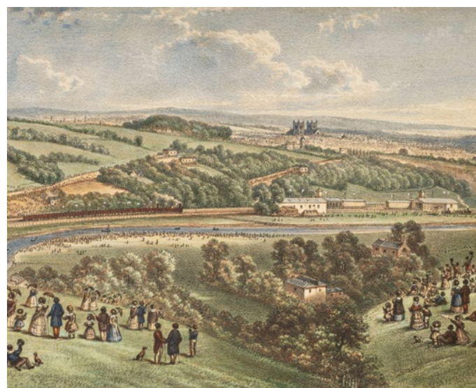
Fig 10 The Opening of the Bristol and Exeter Railway as seen from Exwick Hill in 1844-1850. Painting by W Hake.
