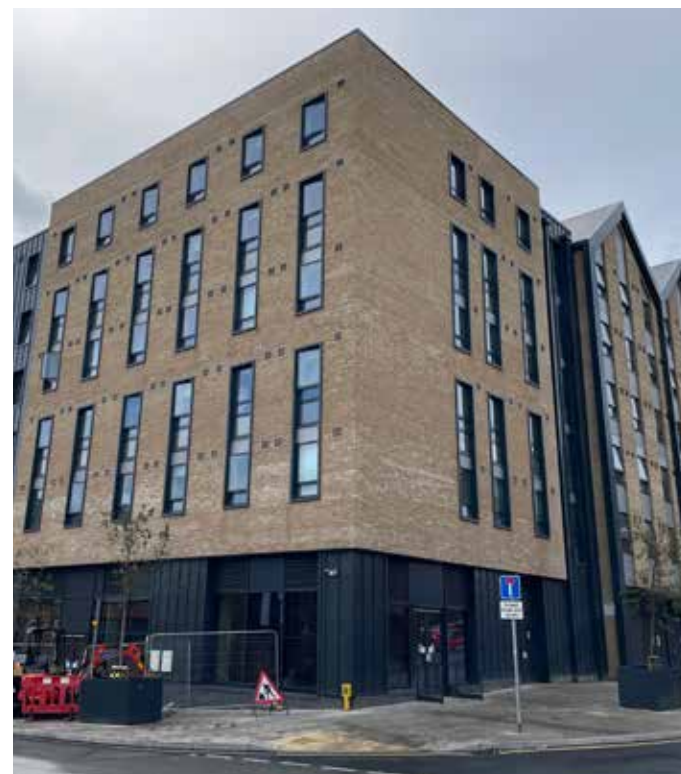
The Depot, Bampfylde Street Brickwork & metal cladding Metal window surrounds
