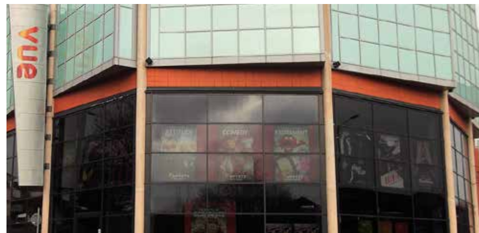
Vue Cinema, Summerland Gate Tile, metal cladding and curtain walling
