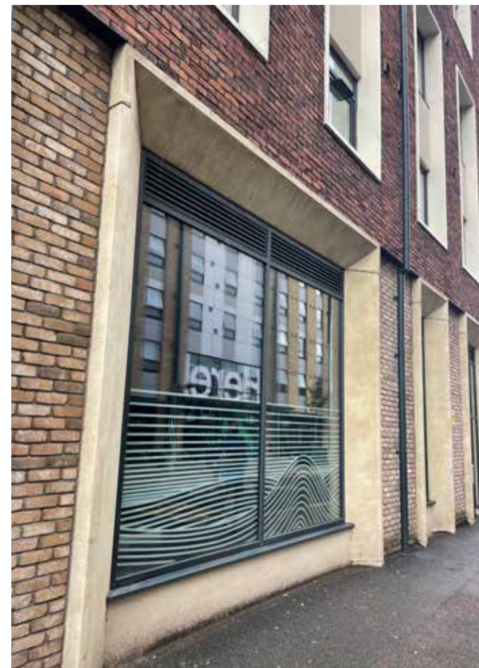
The Barn, Bampfylde Street Palette of brickwork & render Stone window surrounds
