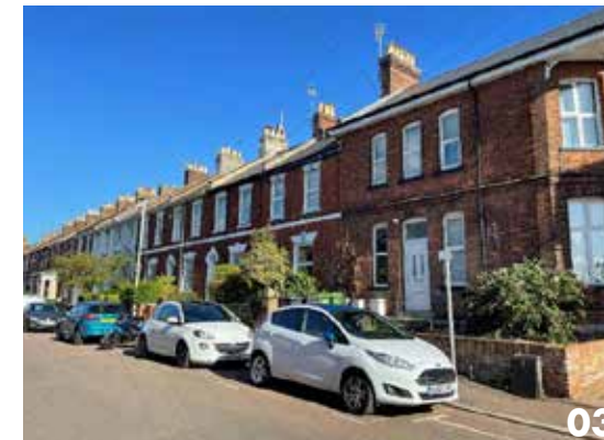
Historic brickwork & slate
