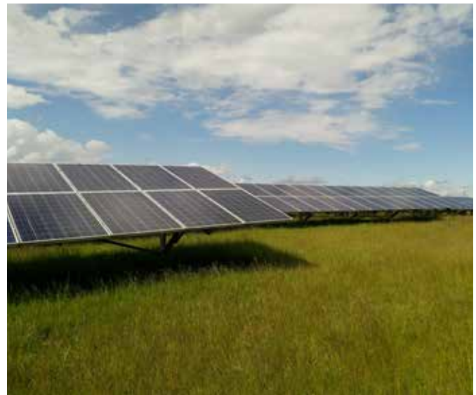
Solar panels in East Devon
