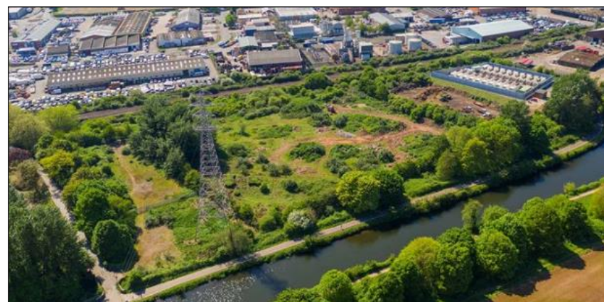
Solar farm and storage project
