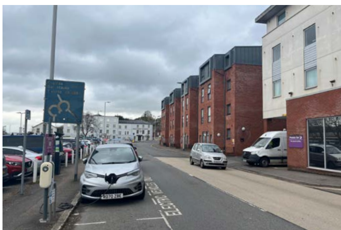
View looking north along Bonhay Road adjacent to station surface car parking
