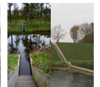
Landmarks crossing of flood channel
