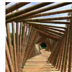
Artistic bridge over water
