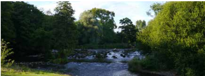
View of Exwick weir
