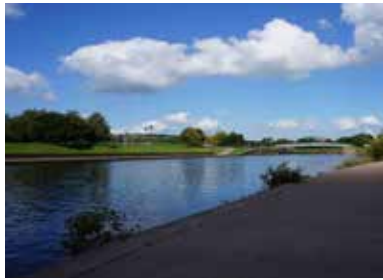
Open view across channel
