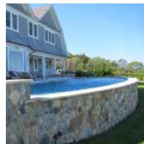
Outdoor swimming pool reinforced with flood wall
