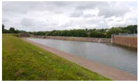
Exwick Spillway and weir
