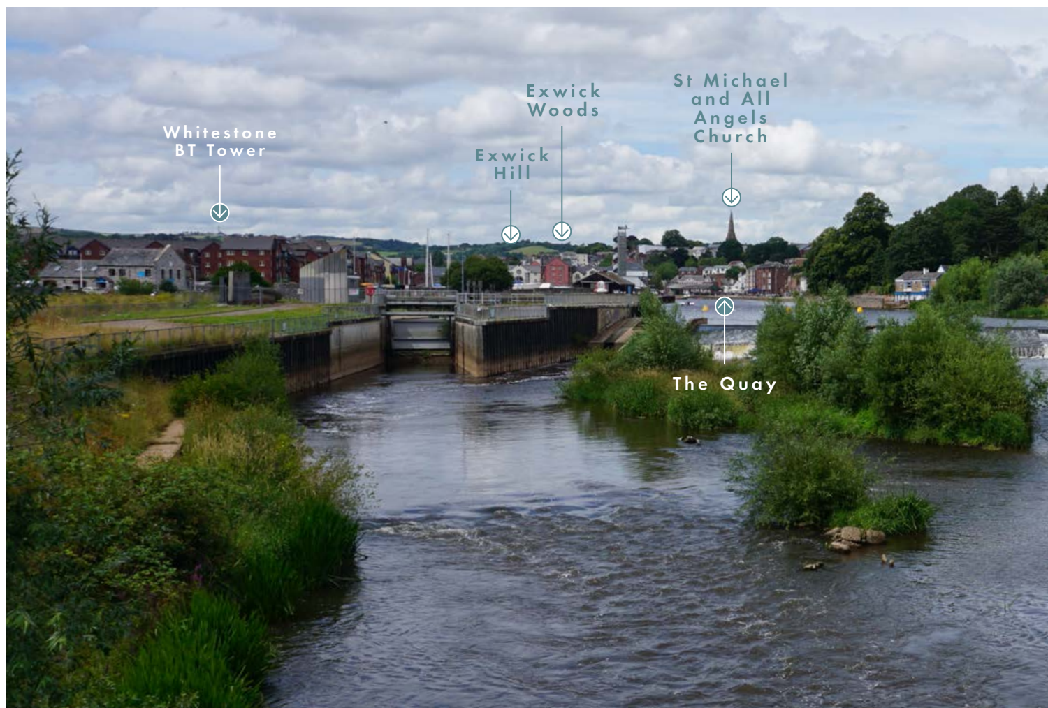
Fig 64 Photo showing R02 Trews Weir Suspension Bridge view towards Exeter City Centre.
