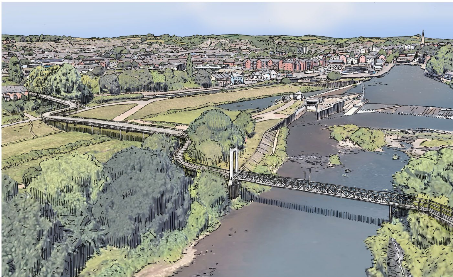
Upstream (north west) view over River Exe
