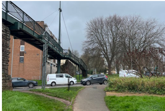
View looking alongside the city wall and pedestrian bridge
