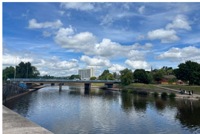
View looking north along River Exe showing Exe Bridge South
