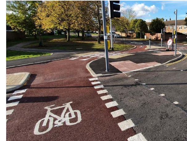
Figure 2: Example of a major junction improvement, Cambridge
