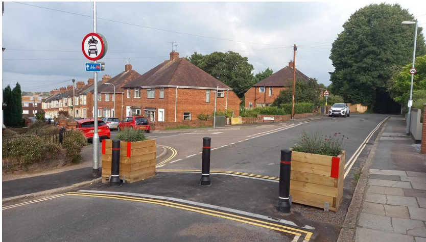
Figure 1: Example of a modal filter, Homefield Road, Exeter
