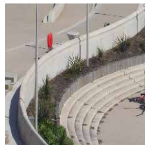
Concrete wall with integrated seating and amphitheatre
