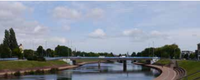
Contemporary Exe Bridges
