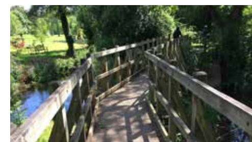
Timber bridge on the Mill Leat
