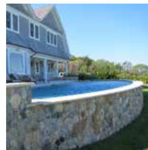
Outdoor swimming pool reinforced with flood wall
