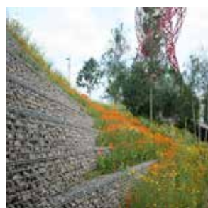
Using gabions can create ecologically sensitive defence
