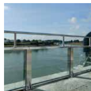
Glass sections of walls improve visibility
