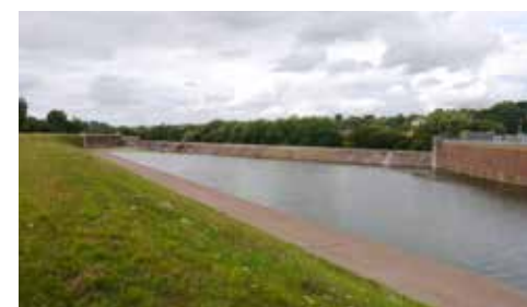
Exwick Spillway and weir
