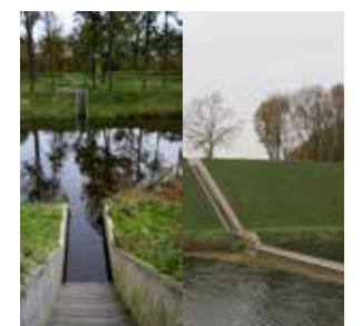
Landmarks crossing of flood channel
