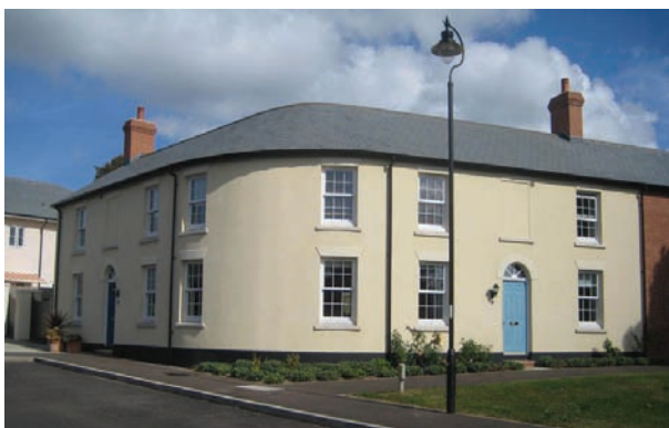
Figure 4.6 Buildings here turn the corner effectively.
