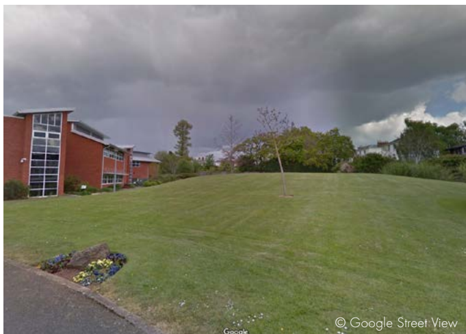
View from north of College House showing green space which backs on to Baring Crescent
