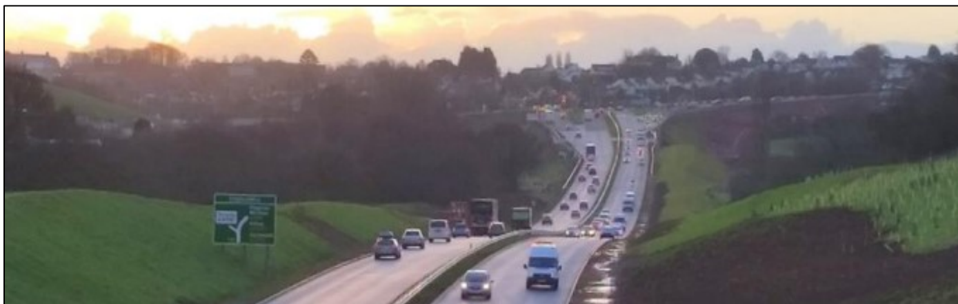
Figure 17: South Devon Link Road completed scheme
