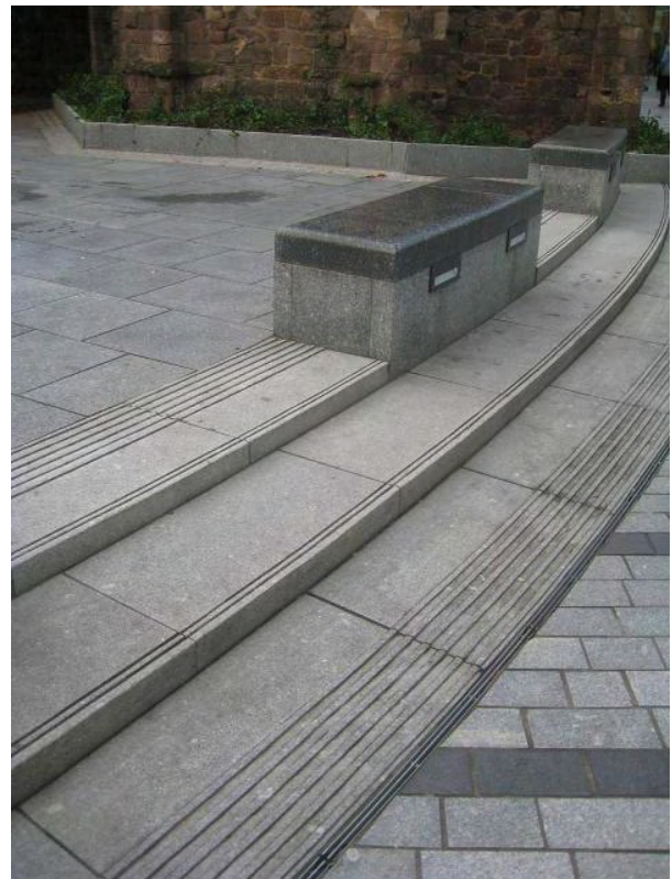
Figure 10.8 Carefully detailed granite steps and tactile paving.
